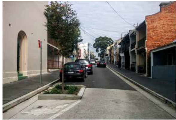
William Street, Paddington: Footpath widening and landscaped kerb blister
